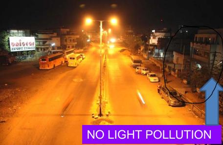
540 W LOAD ON A POLE :42 M SPAN 250 W HPSV LAMP X 2
